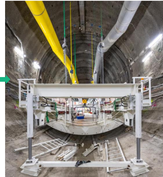
10 m drift lining casting
